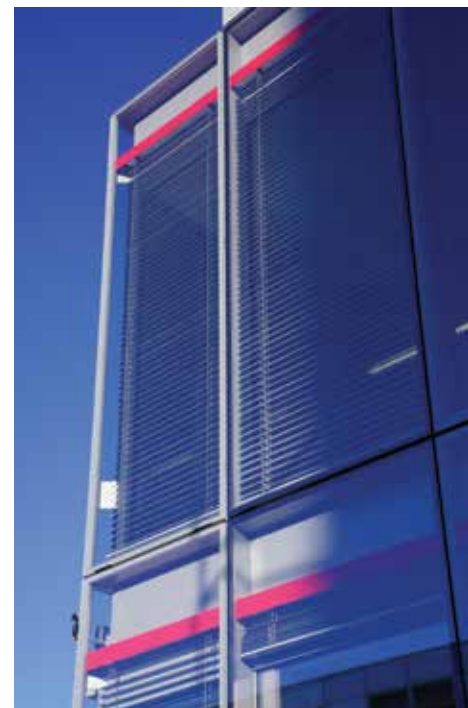
Figure 13. Closed-cavity façade drawings and a photograph of Gartner's visual mock-up unit. © Rob Peebles / PLP Architecture
